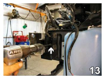
13. Slide the baseplate onto the frame rail and position it as close to the rear of the metal bumper as possible and as high, (toward the top of the frame rail) as possible. Clamp the baseplate to the frame rail using the large vise grips. Using the baseplate as a template, drill three holes in the frame rail with the 13/32" drill bit.
